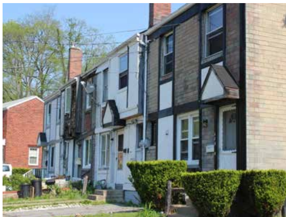
Figure 7: Vacancy and Disrepair
