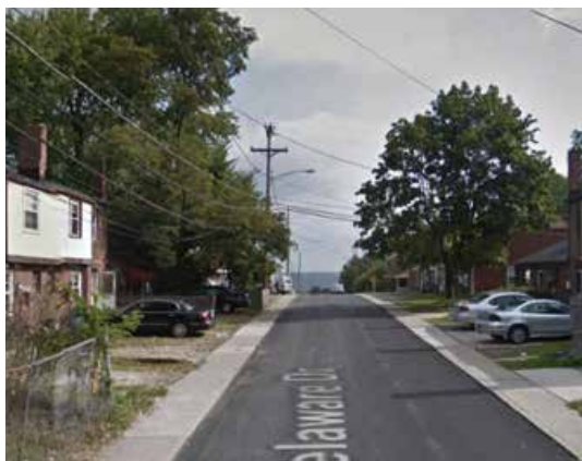
Figure 37: Restore Façades and Remove Fencing
