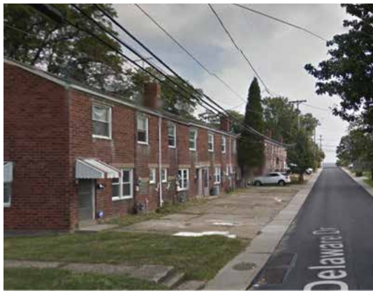
Figure 36: Minor Brick Repairs and Plantings
