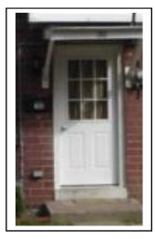
(acceptable) Replacement door The front doors of historic houses are usually consistent with the architectural style of the house. Within the district, solid wood doors with clear glazing in a three over three pane pattern above a lower two paneled area are quite typical.
