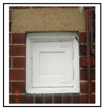
Coal chute door-Note: Lintel is original Must not be not painted
